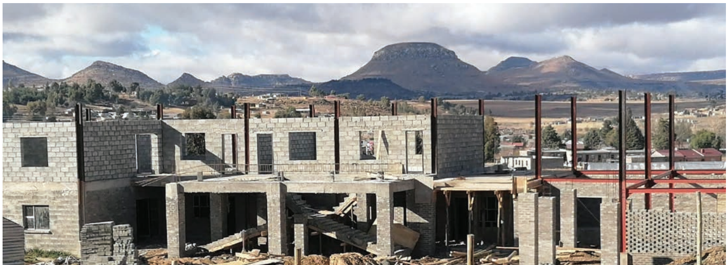
New adjacent center under construction
