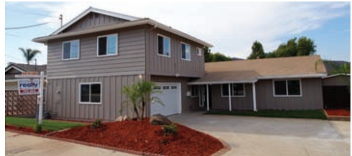
The June Lake house after renovation.
