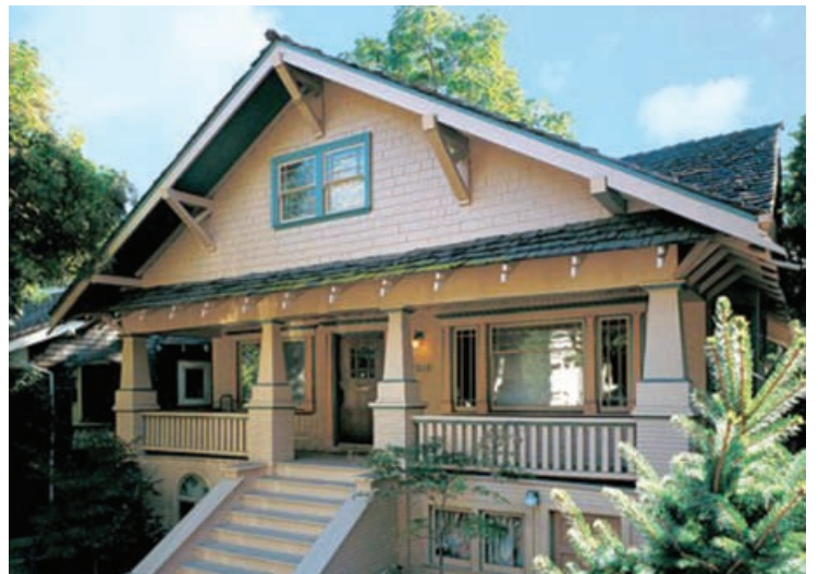
A typical builder’s semi-bungalow with such artistic details as knee-braces under overhanging eaves, exposed rafter tails decoratively sawn, and battered posts on piers. Photo by Douglas Keister.
