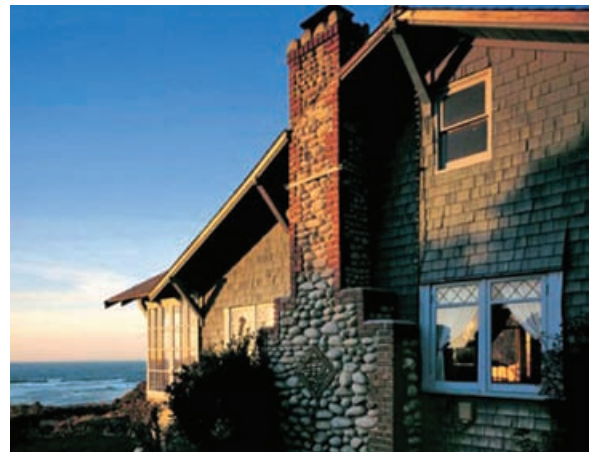
While most often made of wood, bungalows incorporate local materials and vernacular building traditions. Photo by Douglas Keister.
