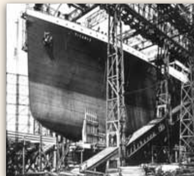
Bow of the Titanic under construction.
