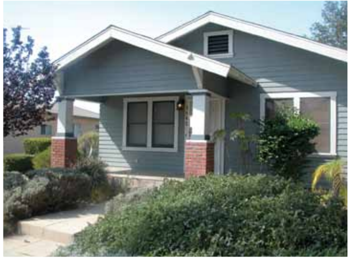
The bungalow at 3642 was built in 1925 and has a one-bedroom cottage in the rear.
